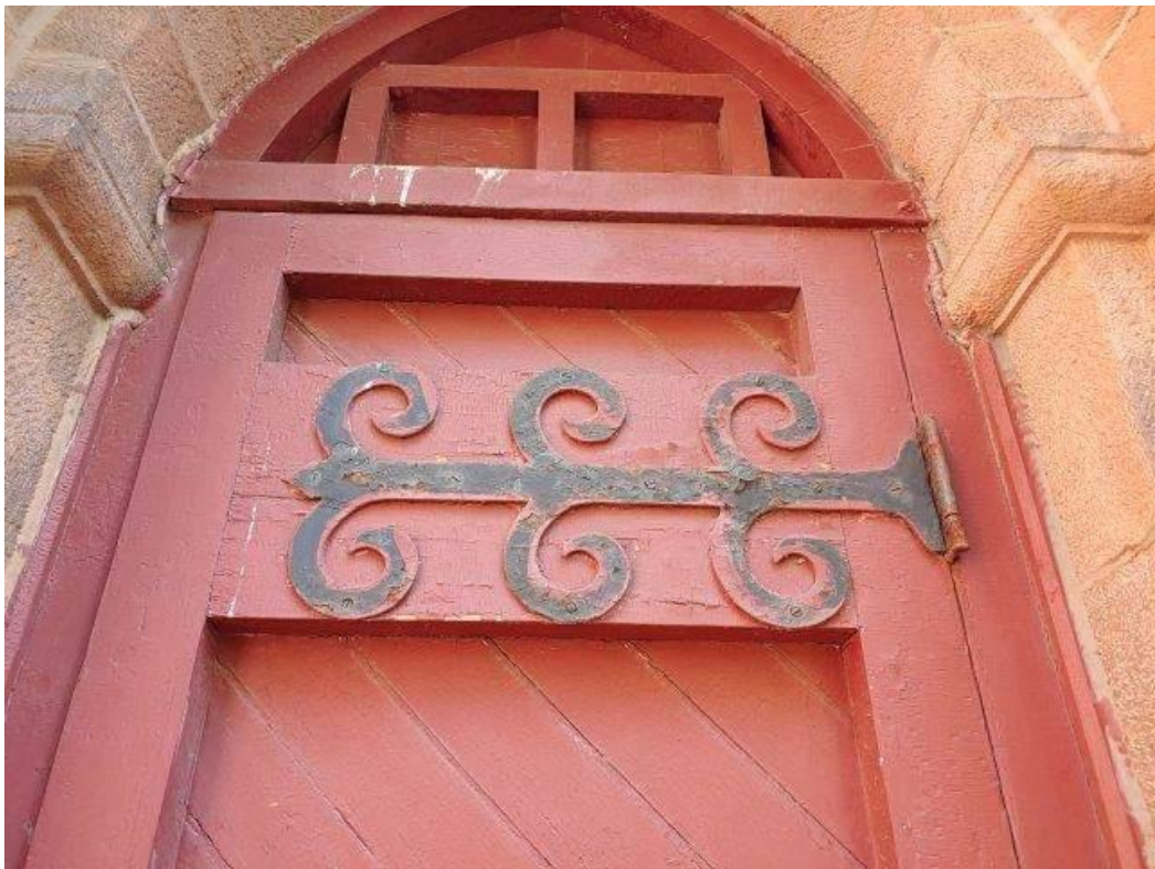
Baptistery Entrance, south door details
